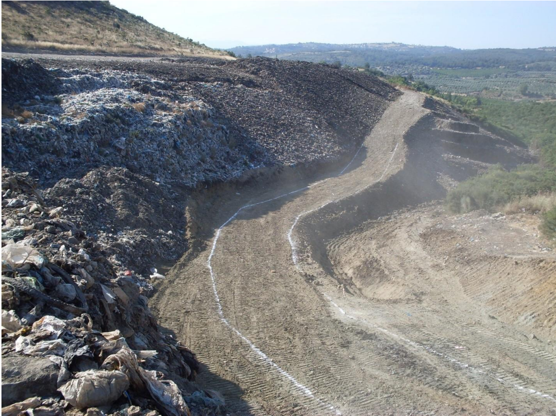
Figure 3.7. Transporting waste inside the border and sloping the area.
