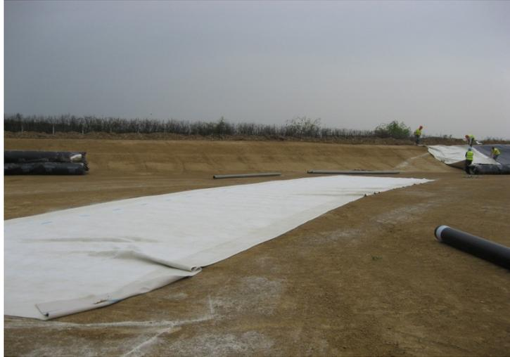
Figure 3. Geomembrane construction of storage cells
