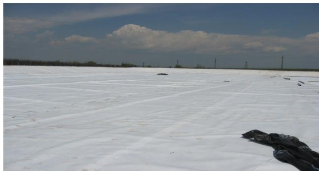
Figure 5. Final cover of storage cells
