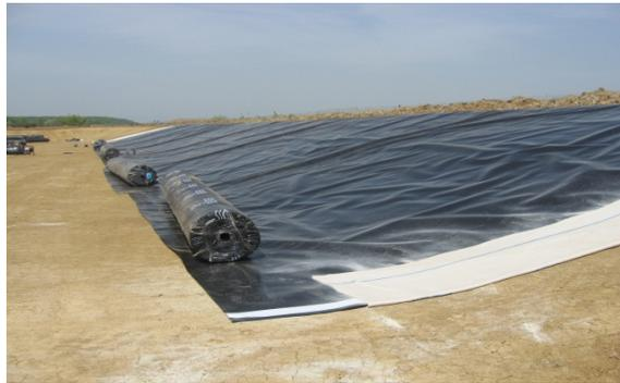
Figure 4. Construction of storage cells
