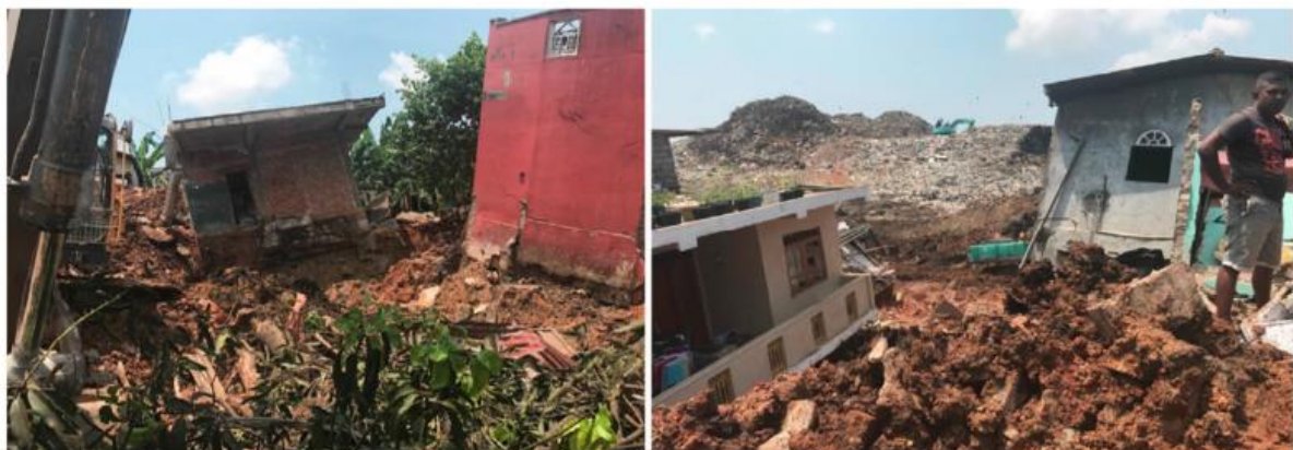
Figure 1.4. Damage to dwelling units because of the slope failure in Meethotamulla open dump (Jayaweera et al., 2019).
