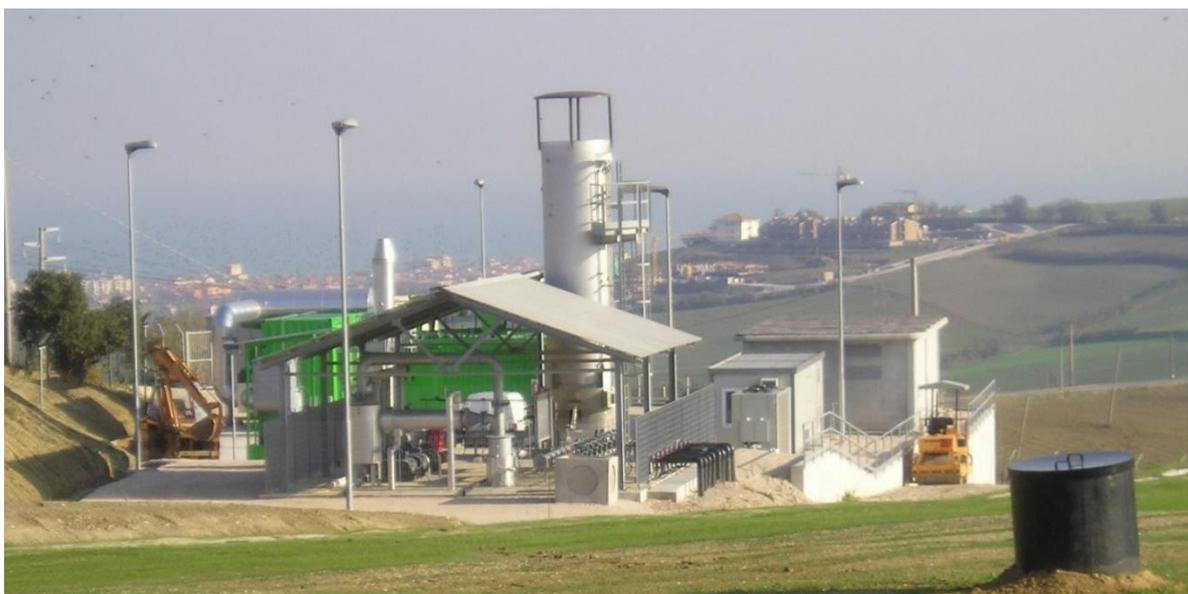
Figure 4.7. Extraction Plant and energy recovery for landfill gas. Source: ASET Spa, 2005.
