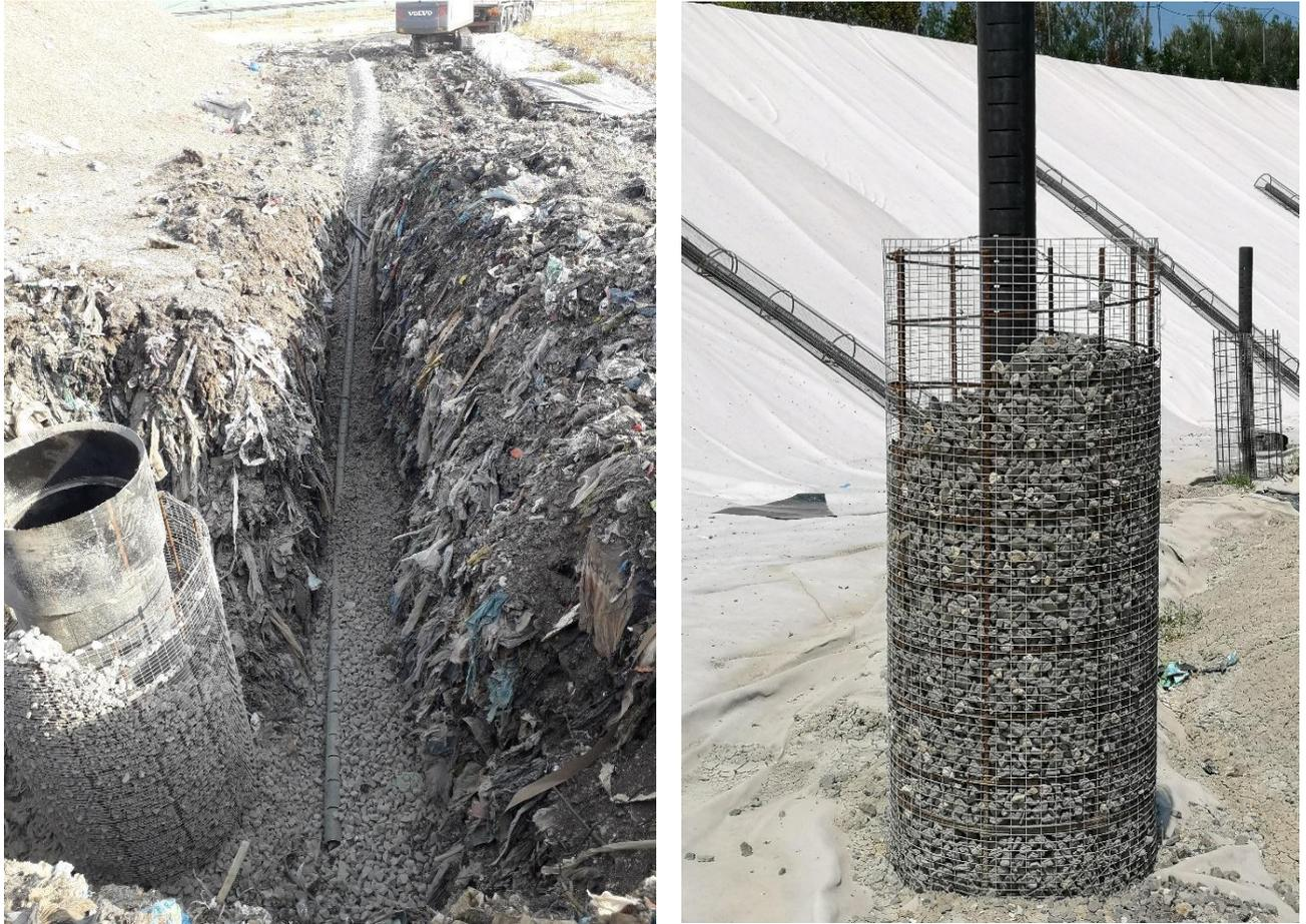
Figure 4.3. Horizontal drainage and wells. Source: ASET Spa, April 2019.
