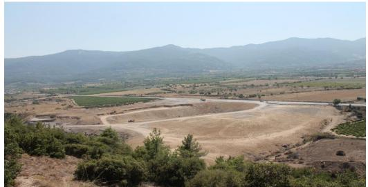
Figure 6. View of the open dump site during top cover formation
