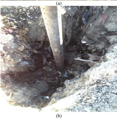
Figure 8. Installation of gas chimney
