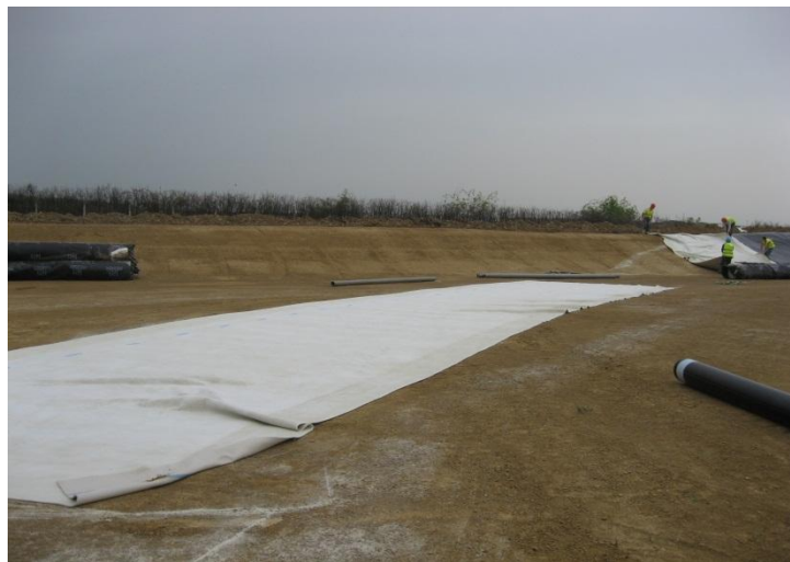
Figura 4. Geomembrane construction of storage cells
