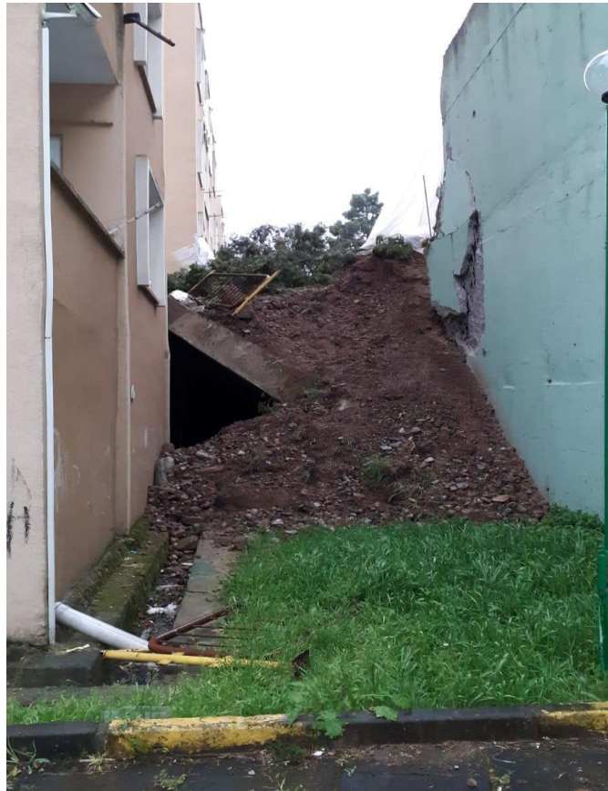
Figure 3.18. Collapsed retaining wall and landslide (or mass movement.)
