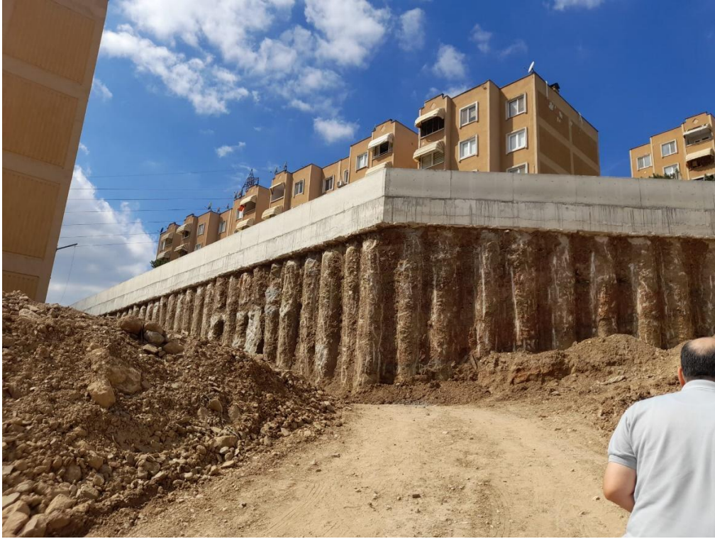
Figure 3.20. Newly built retaining wall.
