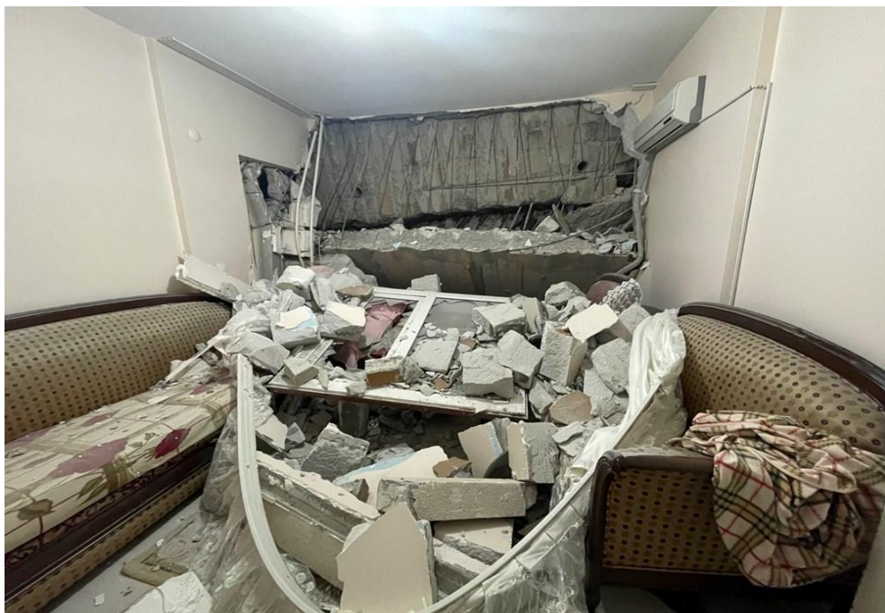
Figure 3.19. A room whose wall collapsed due to the landslide.
