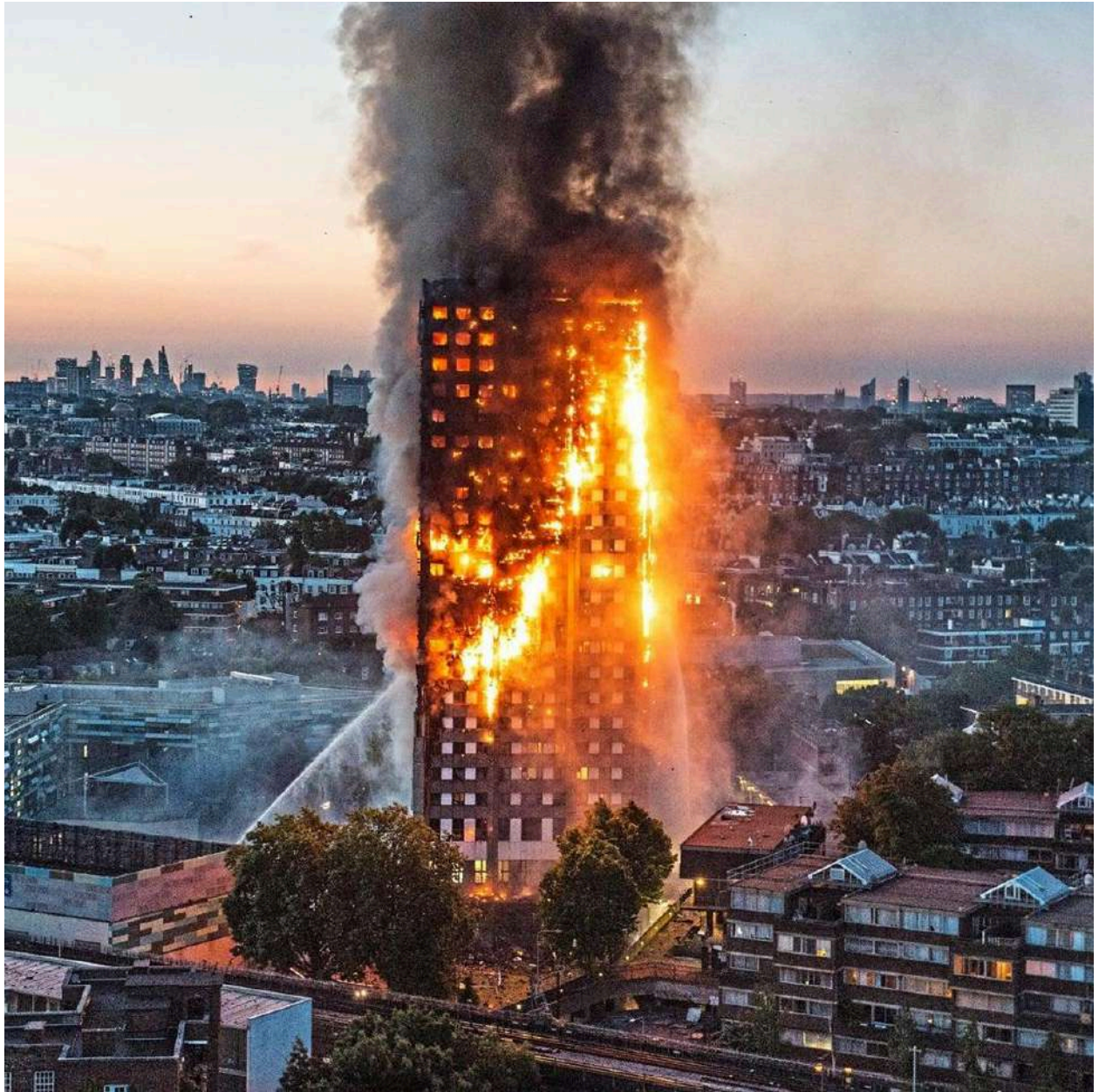
Figure 5.46. Grenfell Tower fire.
