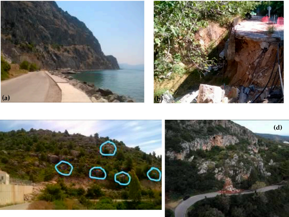
Figure 6.7: (a) Roadside cliff in Attica region, Greece, prone to frequent rockfalls, (b) Chelidonous stream in Kifisia municipality (North of Athens) causes earthfall on bank slopes. (c,d) Spetses and Kithira islands in Attica witnesses rockfalls. The cyan circles are used to emphasize the high likelihood of rockfalls.
