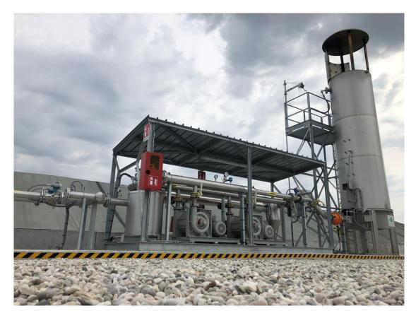
Figure 4.10. High temperature torch. Source: CONVECO Srl,2021. All rights reserved.
