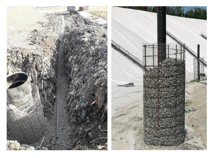
Figure 4.3. Horizontal drainage and wells. Source: ASET Spa, April 2019.
