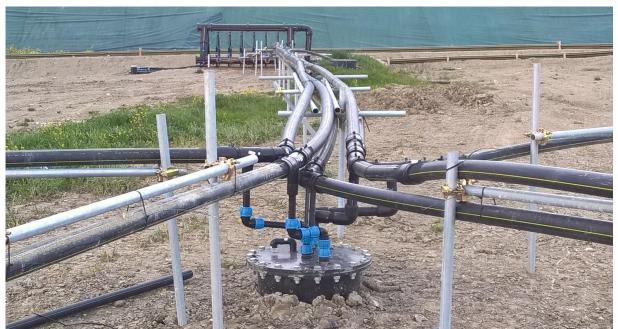
Figure 4.6. Secondary landfill gas lines laid on supports of metal pipes - in the foreground a condensate discharger - in the background a Regulation Station. Source: ASET Spa, Nov.2020.
