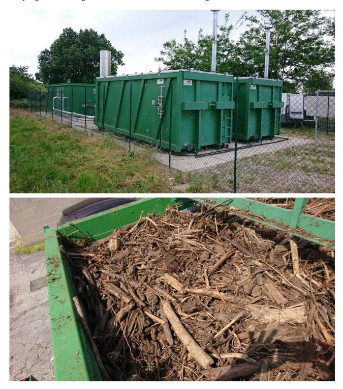
Figure 4.9. Examples of container biofilters with organic material (detail). Source: ASWM Srl, 2021.
